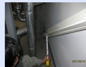
Brace bent by a few centimeters
